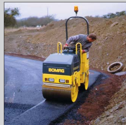
BW 80 AD-2: Operation in restricted conditions; asphalt repairs, car parks
